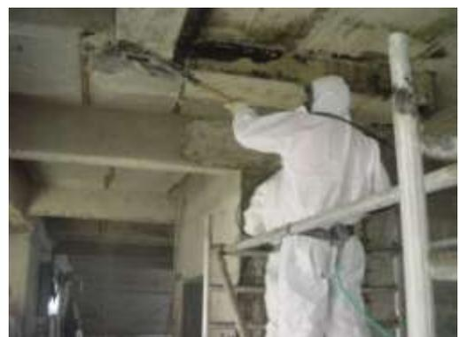
**Figure 2: Sprayed Asbestos removal (Source ETI)**
