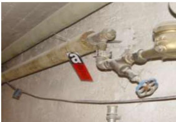
Figure 5: Labelling of asbestos containing materials (Source ETI)
